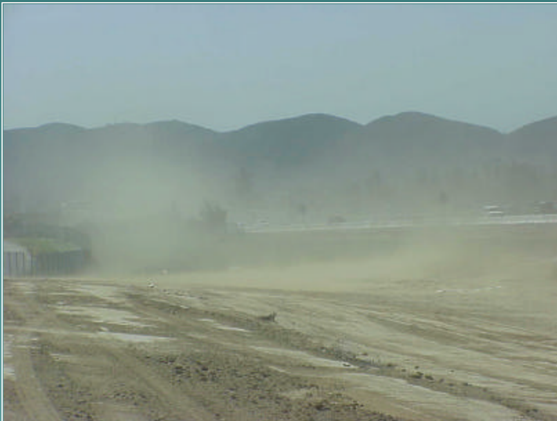
Lack of wind erosion controls
