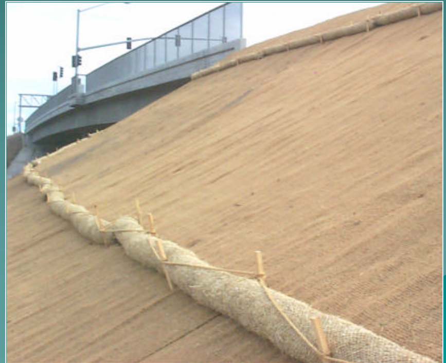
Proper silt fence and fiber roll installation
