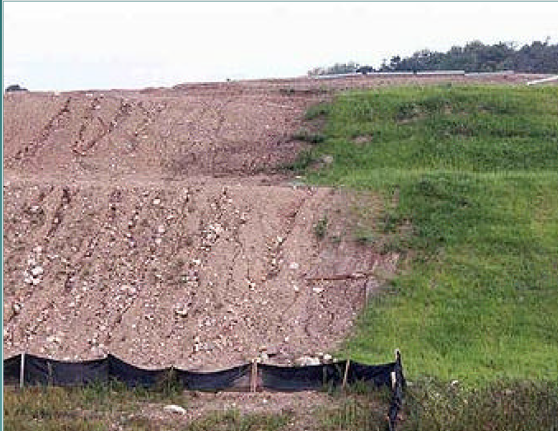
Unstabilized slope vs. Stabilized slope
