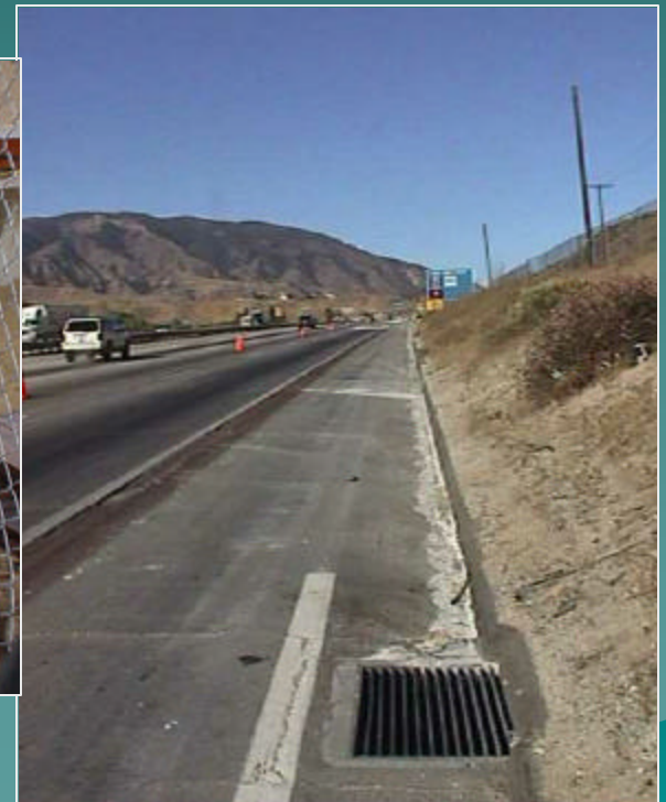
Uncontrolled concrete washouts
